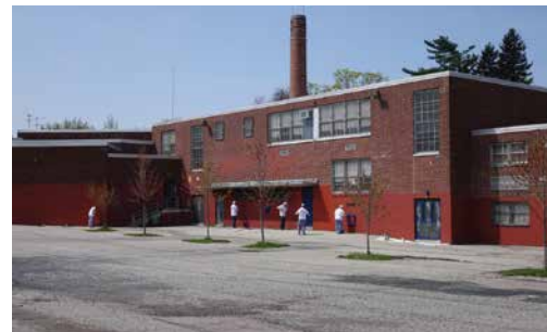
Ellwood Elementary School is located in the Oak Lane section of Philadelphia and is now part of the Fiesta Schoolyards program created by Lindy Communities
